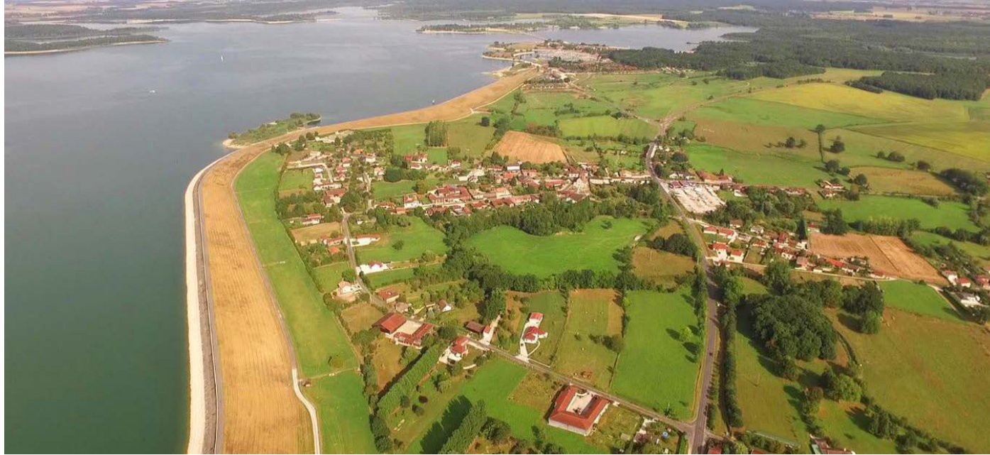
Figure 42: La digue de Guiffaumont
