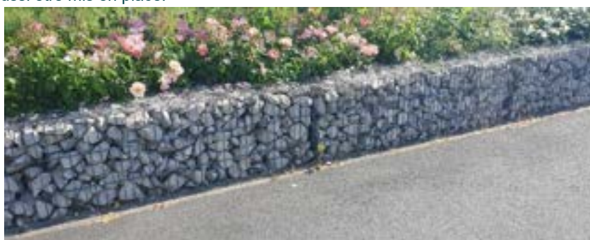
Gabions favorables aux reptiles
