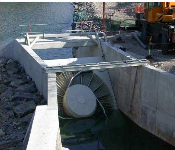
Figure 30 : Turbine VLH de Millau (photo : MJ2 Technologies)
