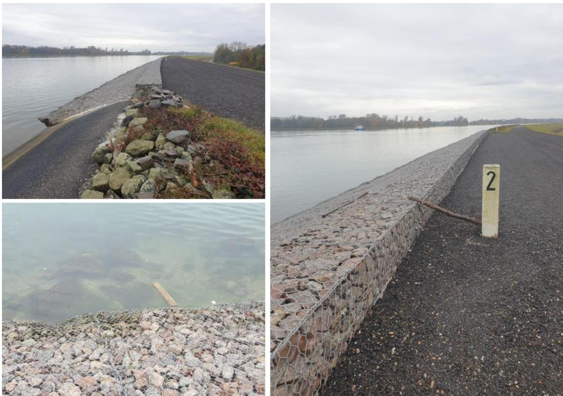
Figure 16 – Parement en matelas gabions
