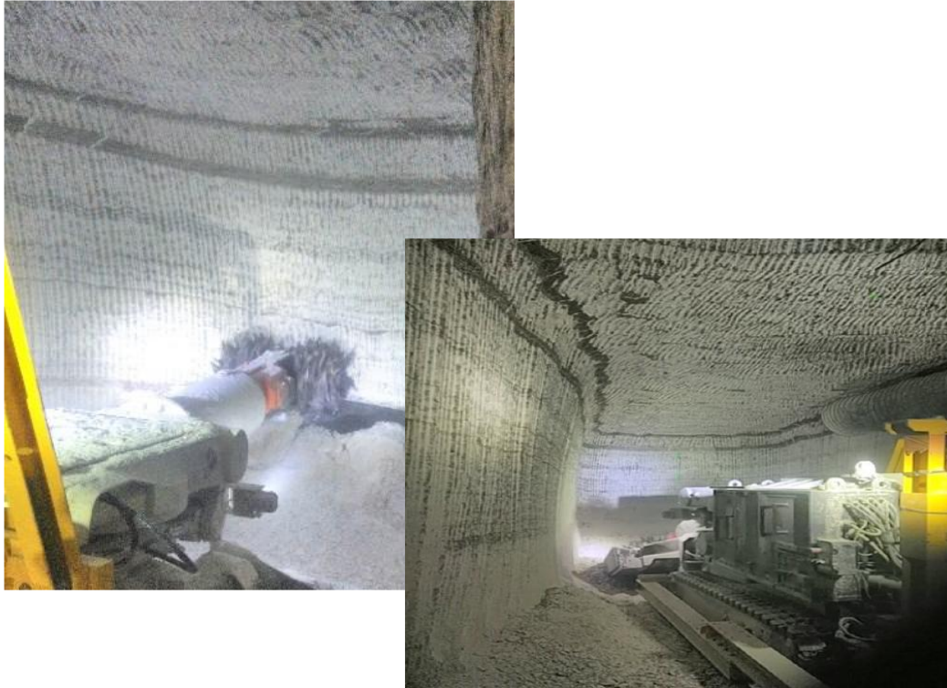
Surexcavation barrage 9b
